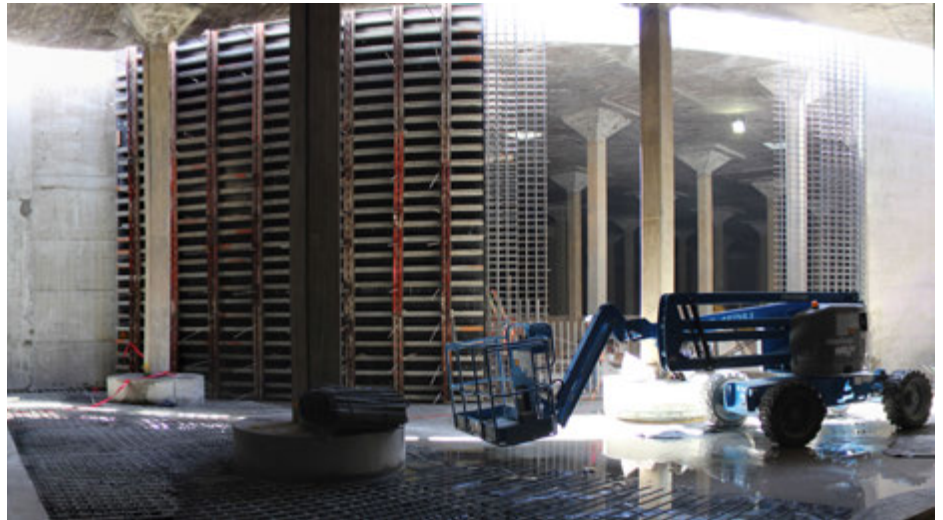
Huntsbury 3 reservoir earthquake recovery work, Christchurch.
