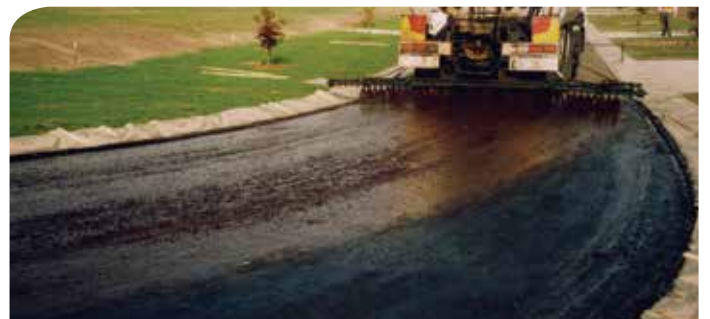
EmulPrime being applied at a premium residential development near the city of Melbourne, Victoria.
