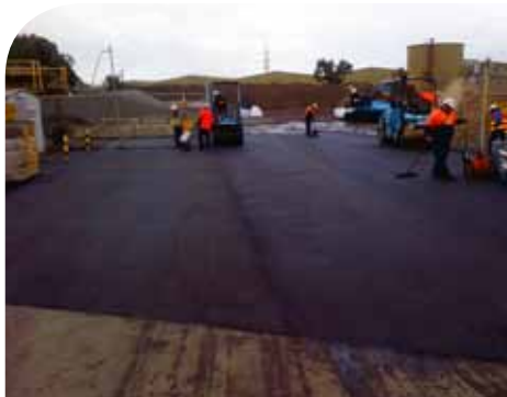
GripPhalt being placed at Westall Asphalt Plant in Clayton South, Victoria.
