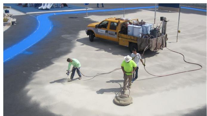
*JetBloc is applied in two even coats in transverse directions.*
