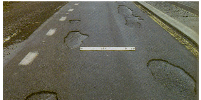
The high tyre pressures and heavy wheel loads from aircraft braking can result in delaminations in pavements constructed with traditional tack coat.
