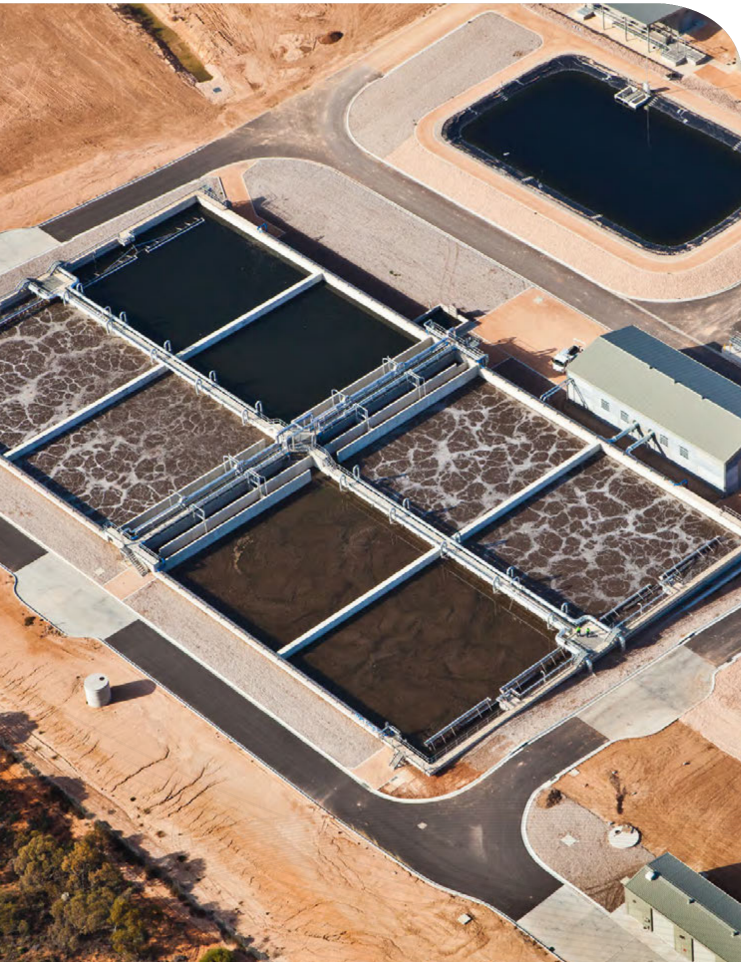
Koorlong Wastewater Treatment Plant, Mildura, Victoria.
