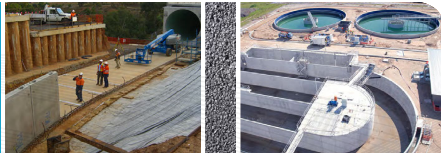
Fulton Hogan has the experience and resources to enter into successful collaborative arrangements, both as a partner and a head contractor.
