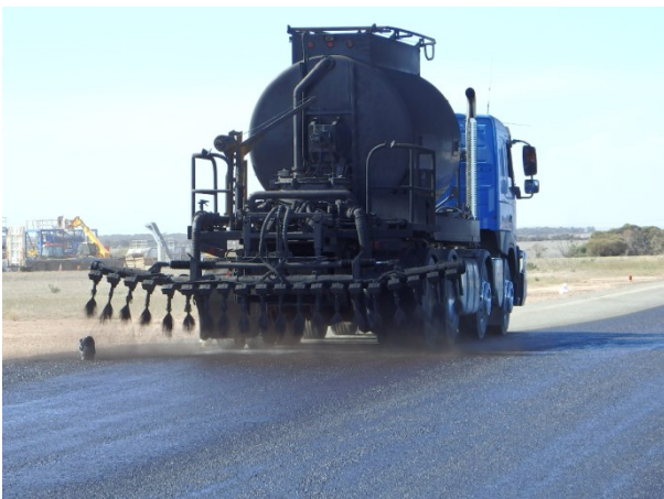
Application of tack coat to an existing pavement.
