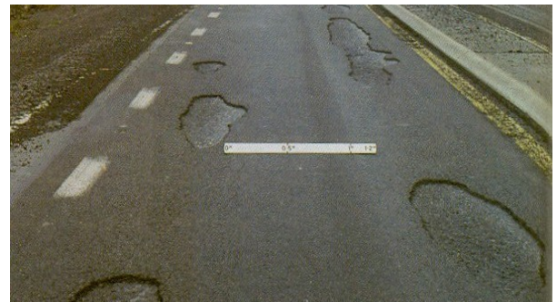
Example of pavement failure: Tracks constructed with regular tack coat can result in pavement delamination due to the extreme pressures inflicted during racing.
