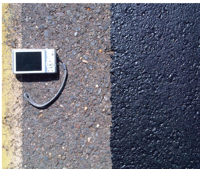
Side by side comparison of aged asphalt before and after JetBlack application.
