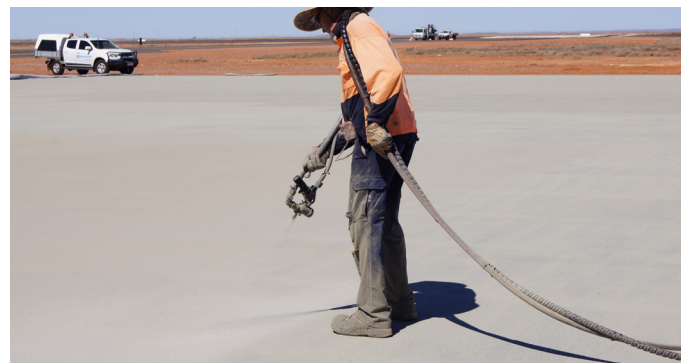
JetBloc is applied in two even coats in transverse directions.
