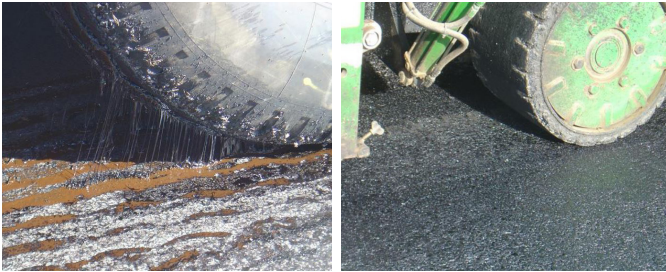
Pick up on tyres with conventional tack coat.
